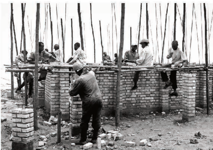
Gikomero ECD construction - local materials and technology
